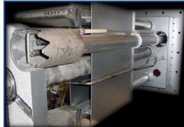
Fyr-Bolt Igniter for a T-fired Boiler
